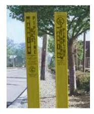
The markers display the material transported in the pipeline, the name of the pipeline operator and a telephone number where the pipeline operator can be reached in the event of an emergency.
