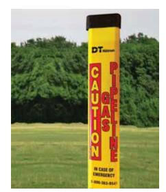
Please remember... before you break ground, Pennsylvania law requires that you call 811 or contact PA-One Call System at least three working days in advance to have the location of underground pipelines marked. Natural gas pipelines will be marked with yellow paint, flags or stakes. You can also contact PA-One Call System by dialing 800-242-1776. It's FAST, It's Free, and it's the LAW.
